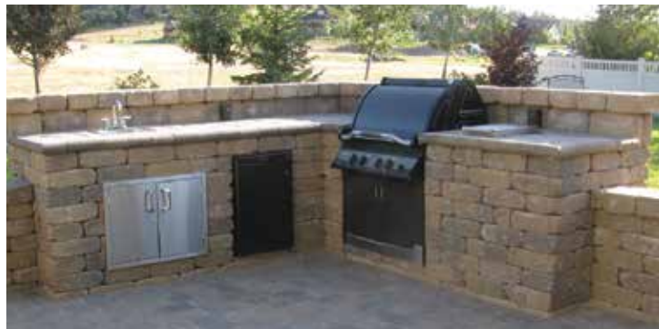
Photo of an outdoor kitchen in progress by Outdoor Expressions in Billings, MT.
